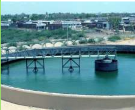
Waste water management
